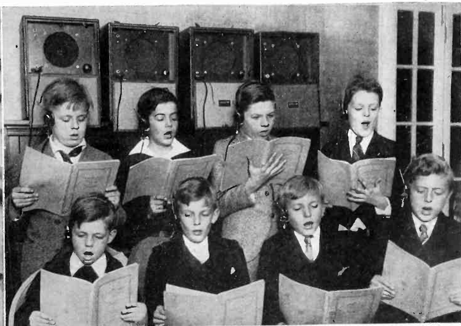
The photocells used for four-part choral instruction. The film containing sound tracks for the separate parts is scanned by individual photocells. The boys in the Electro Choir follow the music they hear in the earphones. Their voices, picked up by microphone, are blended with those of the three other groups singing the other parts
